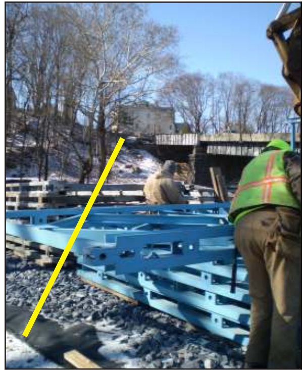
The pedestrian walkway will be at a 10% grade similar to the current sidewalk. In photos the yellow line represents the placement of the walk.
